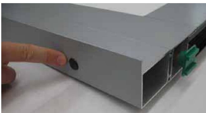
6.24 Close the visible holes with the supplied caps, as shown in the diagram.
