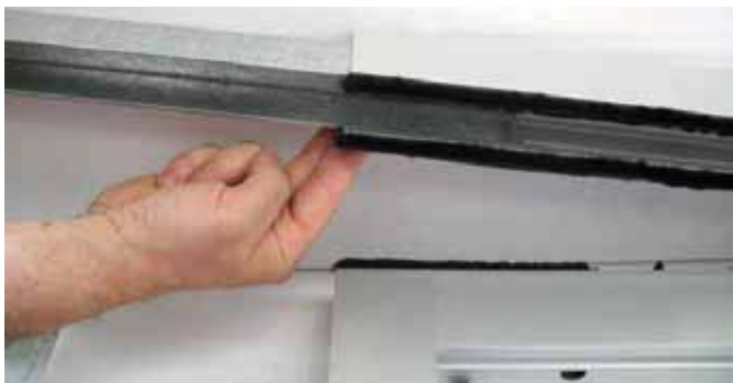
1.16 If the width of the mobile wing is greater than 1000 mm, insert reinforcement 4173 into profile 3820, as shown in the diagram.
