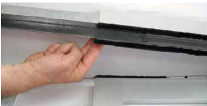
6.16 If the width of the mobile wing is greater than 1000 mm, insert reinforcement 4173 into profile 3820, as shown in the diagram.
