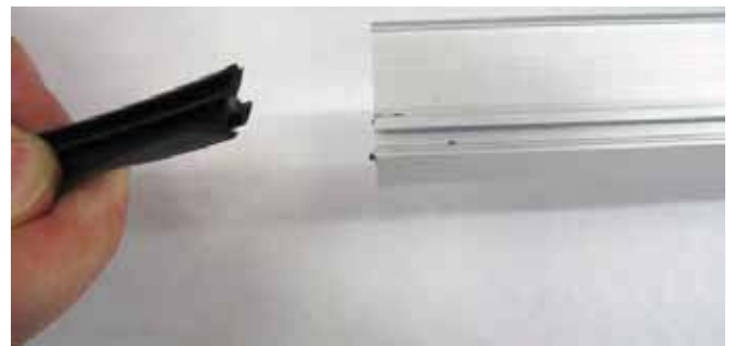
4.26 With PAM45M profiles, insert the seals into the glass-blocking profiles [8], as shown in the diagram.
