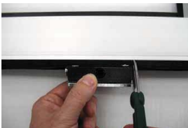
6.13 Trim the brush SPA4811 where it connects with detail [5], as shown in the diagram. Note: Be sure to take note of the wing's opening direction.
