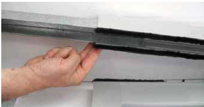
4.16 If the width of the mobile wing is greater than 1000 mm, insert reinforcement 4173 into profile 3820, as shown in the diagram.
