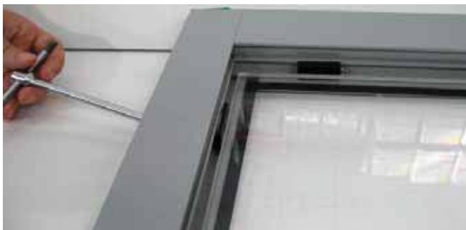
2.26 With PAM45M profiles, insert the glass [9] into the fixed wing, as shown in the diagram.
