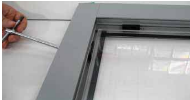
6.25 With PAM45M profiles, insert the glass [9] into the mobile wing, as shown in the diagram.
