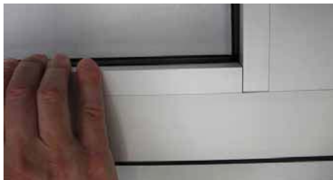
1.29 With PAM45M profiles, insert the glass-blocking profiles [8] onto the mobile wing until they click, as shown in the diagram.
