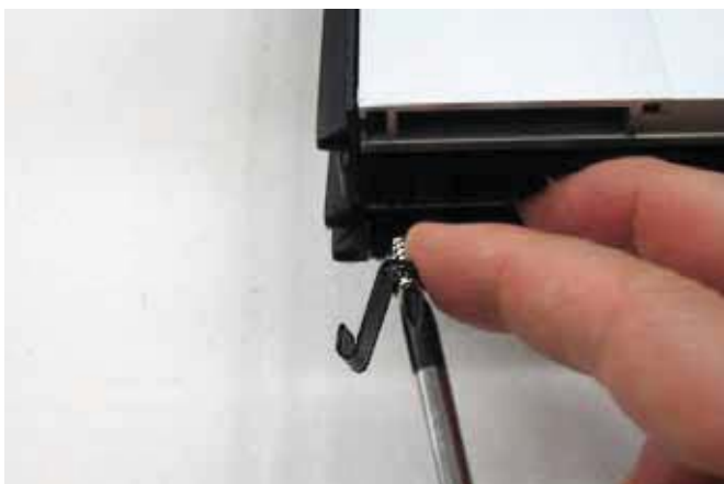
1.22 Attach the supplied hook to the lower part of the wing, as shown in the diagram, in order to prevent seal 3837 from sliding.
