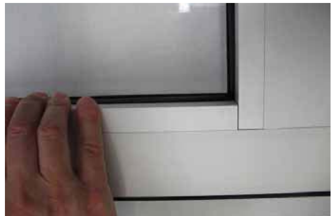
4.27 With PAM45M profiles, insert the glass-blocking profiles [8] onto the mobile wing until they click, as shown in the diagram.
