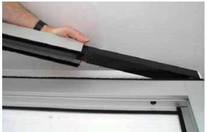
1.14 Insert profile 3820 into detail [3], as shown in the diagram.
