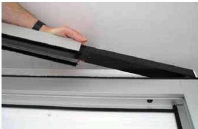
6.14 Insert profile 3820 into detail [3], as shown in the diagram.
