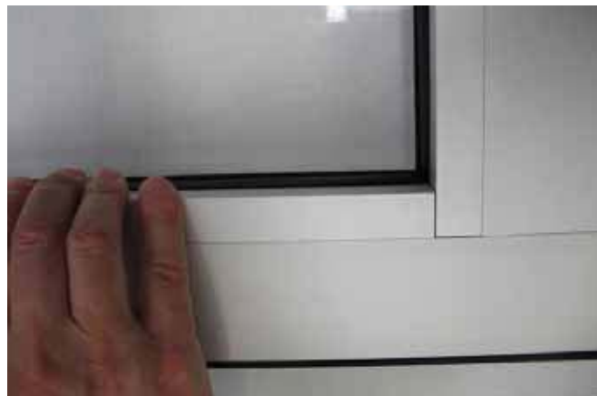
2.29 With PAM45M profiles, insert the glass-blocking profiles [8] onto the mobile wing until they click, as shown in the diagram.
