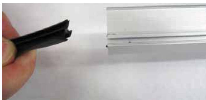
1.28 With PAM45M profiles, insert the seals into the glass-blocking profiles [8], as shown in the diagram.
