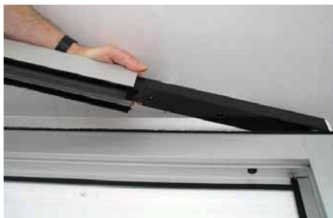
4.14 Insert profile 3820 into detail [3], as shown in the diagram.
