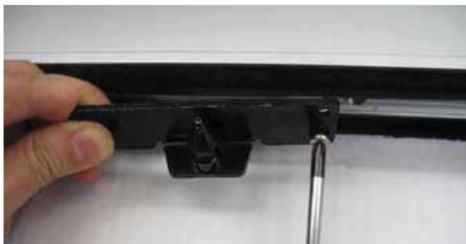
6.12 Fasten detail [4] to profile 3924, as shown in the diagram. Note: Be sure to take note of the wing's opening direction.
