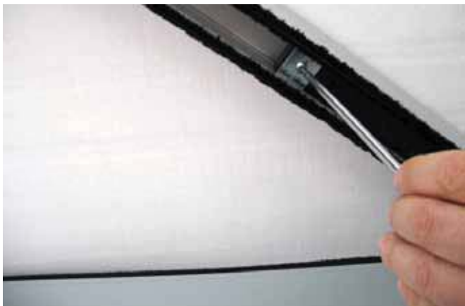
Note: during the installation of the fixture, in order to obtain the proper horizontal position of the mobile panic wing, loosen the fastening screws and adjust the screw shown in detail [3], as shown in the diagram.
