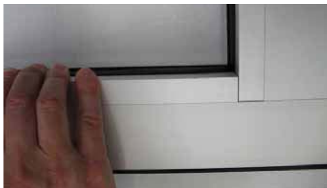
6.28 With PAM45M profiles, insert the glass-blocking profiles [8] onto the mobile wing until they click, as shown in the diagram.
