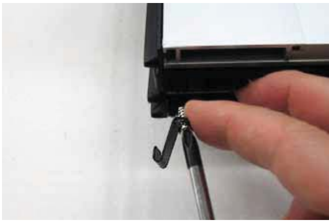
4.22 Attach the supplied hook to the lower part of the wing, as shown in the diagram, in order to prevent seal 3837 from sliding.
