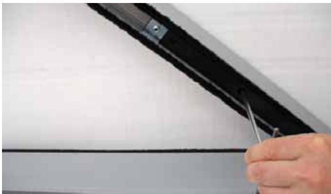
1.15 Fasten detail [3] to profile 3820, as shown in the diagram.
